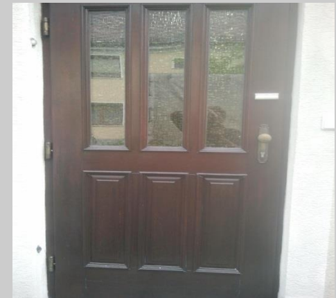
after being coated with KaWaTech
